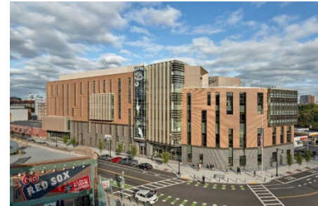
Boston Arts Academy, which opened in September 2022, is 100% electric and is targeting LEED gold certification.
