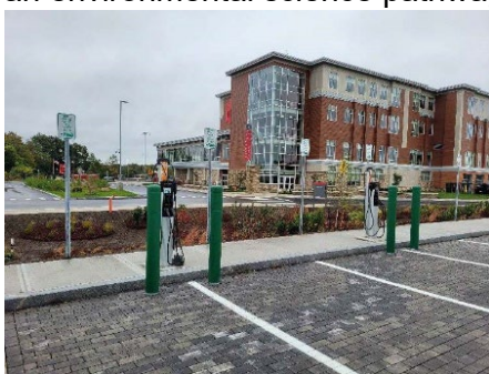
East Providence High School features electric car charging stations and permeable pavers in the parking lot.
