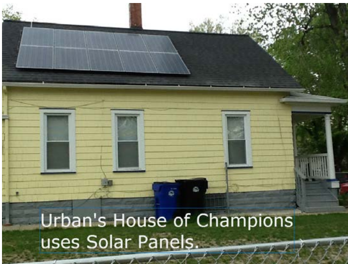
Solar panels (installed spring 2015)
