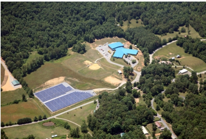
Martins Creek Elementary School – Solar Array Photo credit: ESA Renewables, LLC
