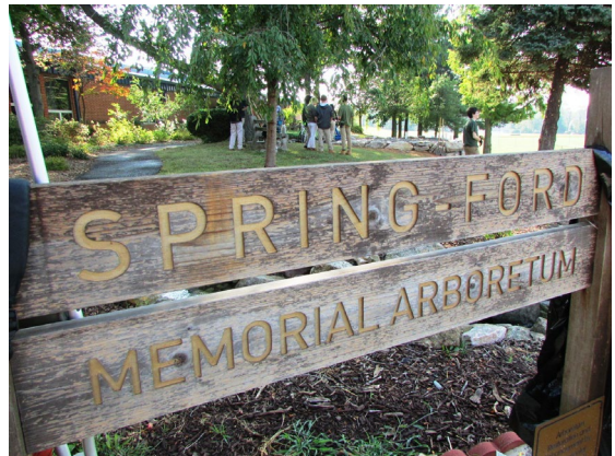
Under the guidance of industry professionals, Spring-Ford Area School District students designed and constructed improvements to the district's arboretum as well as a courtyard area.
