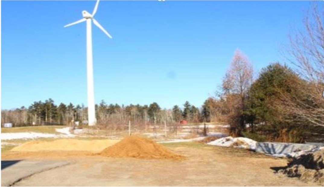
Camden Hills Regional High School's student group, the Windplanners, spearheaded an effort to install a 100-kW wind turbine and a 159-kW solar array. These two installations provide 30 percent of electricity needs from on-site renewable energy.
